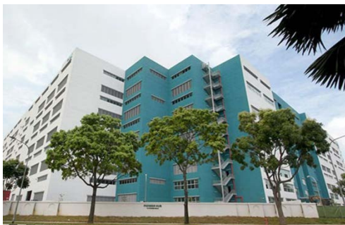
Equinix Singapore 2012 - ongoing
