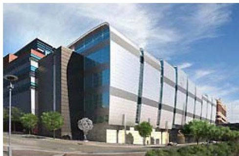
Global Switch Australia 2012 - ongoing
