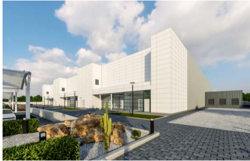
Khazna Data Center United Arab Emirates 2012 - ongoing
