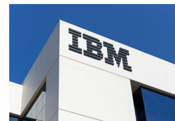
IBM Data Center, Spain
