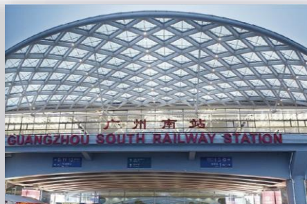
Guangzhou South Railway Station
