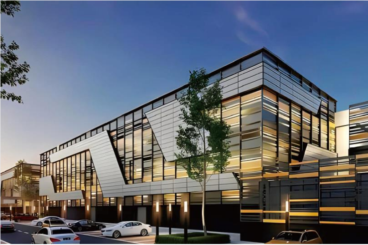
Malaysia Johor MY06 Data Center
